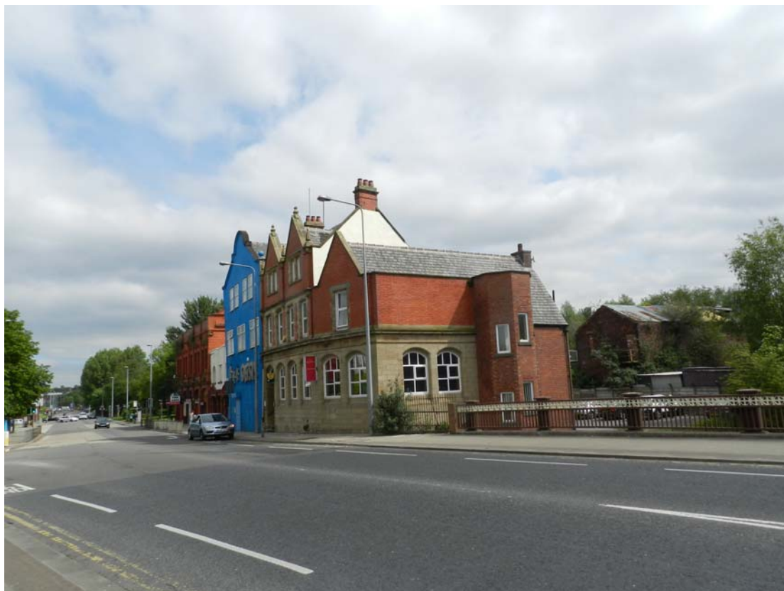
OLD BANK BUILDING, 6 GREAT CLOWES STREET, LOWER BROUGHTON, SALFORD, M7 1RE
